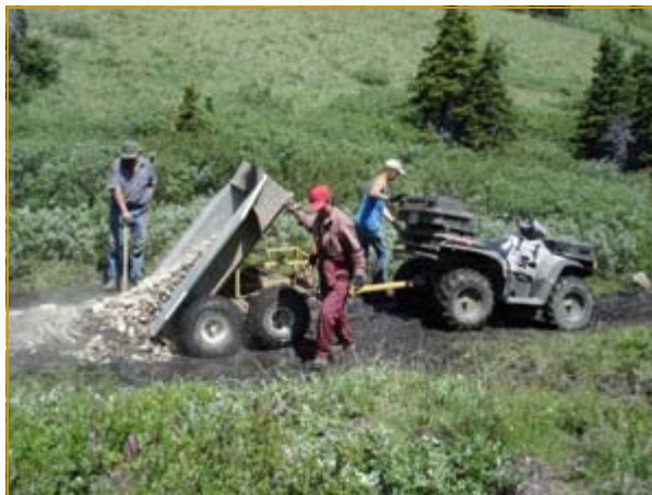
Hauling gravel to repair soft spots in low lying areas
